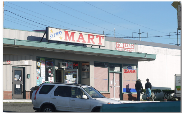
Skyway Mart. Located in the commercial area of the neighborhood just south of the proposed site. Source: C.S. Fowler Consulting LLC.
